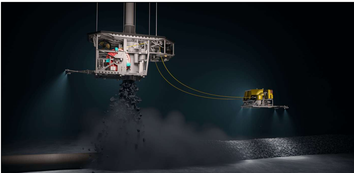
Figure 10: Fall Pipe Discharging Rock
